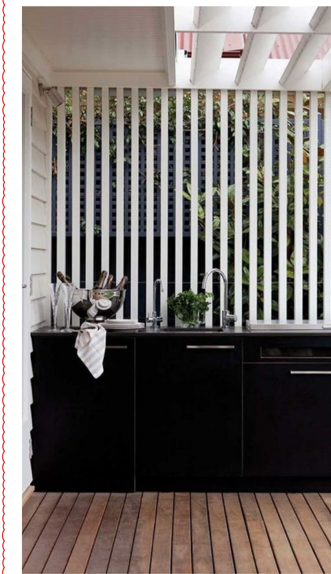
PRIVACY SCREENS TO REAR GROUND FLOOR ALFRESCO SPACES & FRONT FACADE FIRST FLOOR BALCONIES TIMBER POSTS WITH MAX 30MM GAP BETWEEN POSTS TO COMPLY WITH SEPP CLAUSE 1.5
