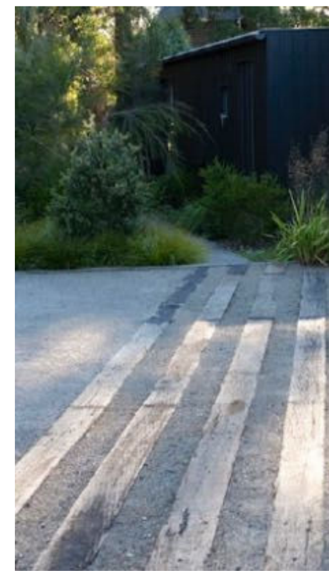
PERMEABLE DRIVEWAY RECYCLED SLEEPERS WITH PEBBLES
