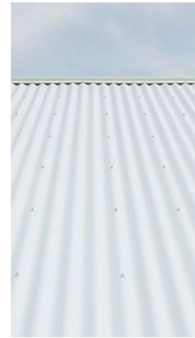
MR.01 METAL ROOF COLORBOND DOVER WHITE
